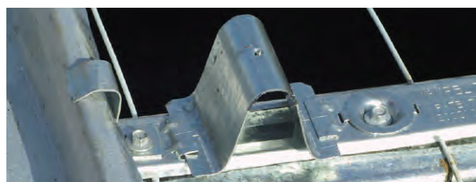
ClearSlide decking support ready to be crimped to deck.
